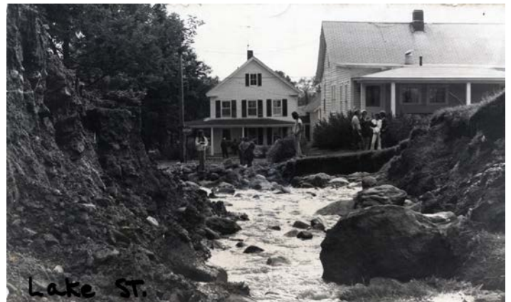
Road washout from 1973 Flooding
