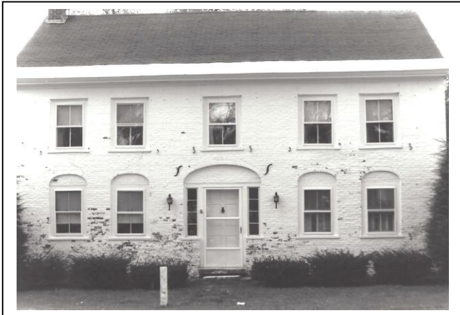
Brick Home as it looks today
